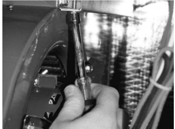
Removing the Supply Blower
